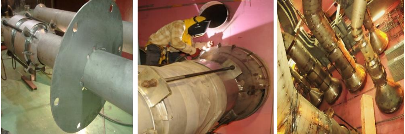
Figure-5: Sodium pipe penetration in RCB wall
